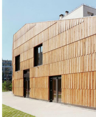
Christian Marin Community Center / Guillaume Ramillien Architecture
